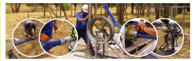
Light and flexible polyurethane layflat hose with drinking water approval, designed as a permanent alternative to traditional materials in water wells with electric submersible pumps, manufactured in Norway to exacting standards.
